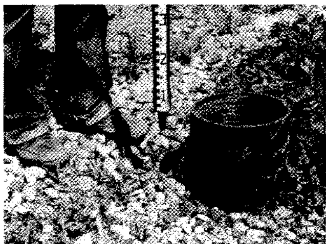
Figure 10. Well casing monument. Rod welded to casing provides a "deep" monument (to depth of cement bond) for the cost of a field weld. Rod is long enough to clear wellhead or wellhead piping. Note upward slope eliminates need for decision or possible inaccuracy in selecting location on a rod set level or near level.
